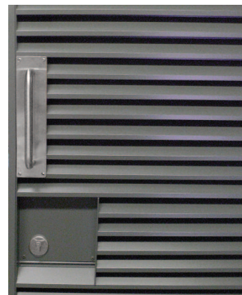
Typical lock and handle arrangement
